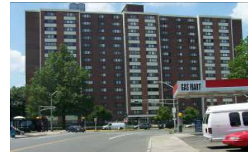
Brookside Apartments, 777 Springdale Avenue
